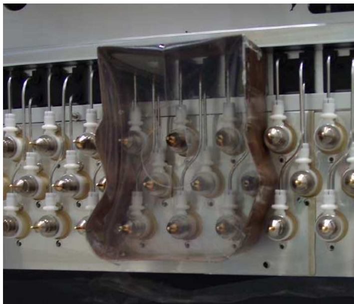
Figure 2: Mask used to localize the leak search.
